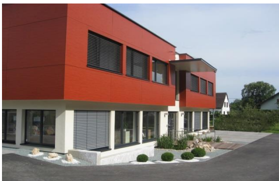
Fig. 8: Façade cladding using compact laminates
