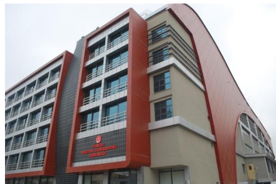
Fig. 8: Façade cladding using compact laminates
